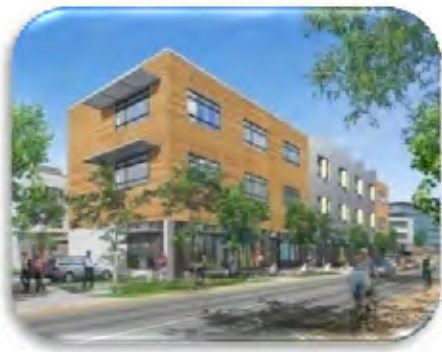
CI-2 Prosperity (under construction)
